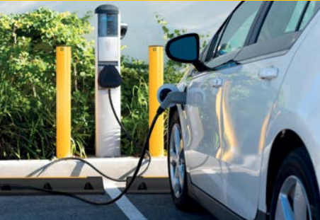
Bollards protecting electric car charging point.
