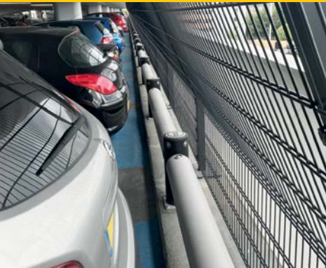
iFlex Single Traffic High Level guarding boundaries in a multi-level parking lot.
